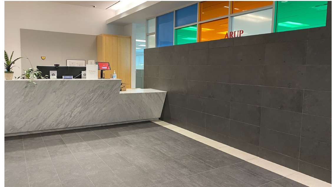
After (complete; removed, not replacing)
